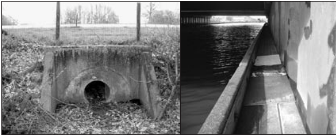
Stubwall under viaduct
